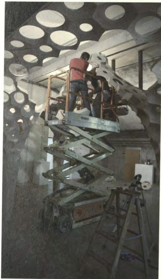
拱的组装 Assembly of the vault
