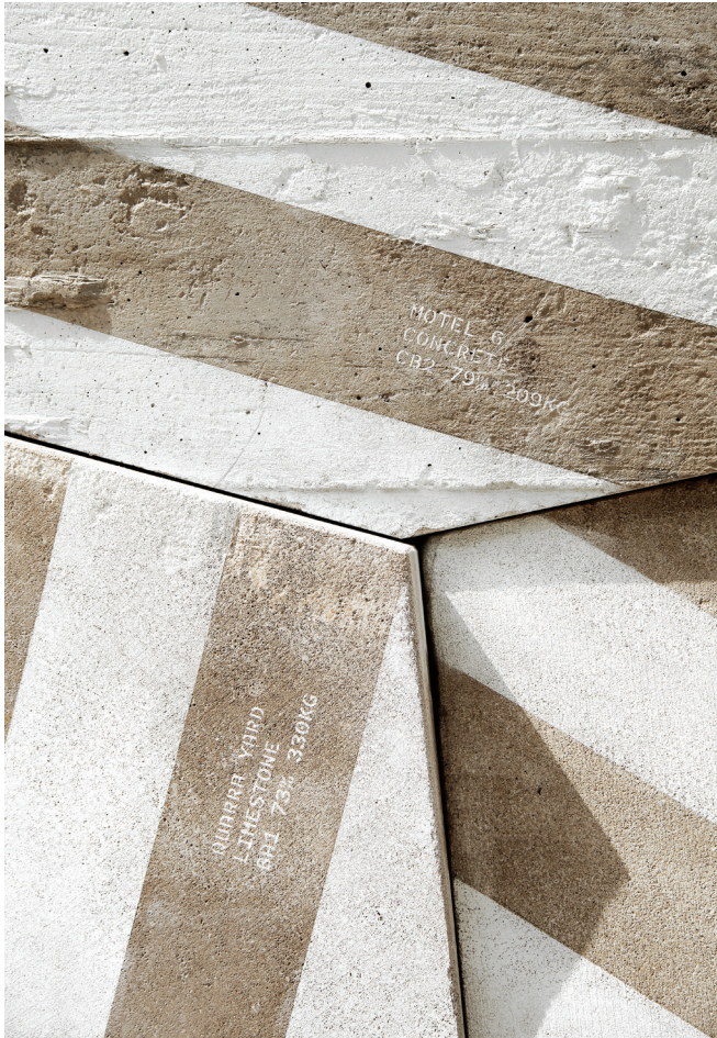
18 Detail of the back side of the wall assembly.
