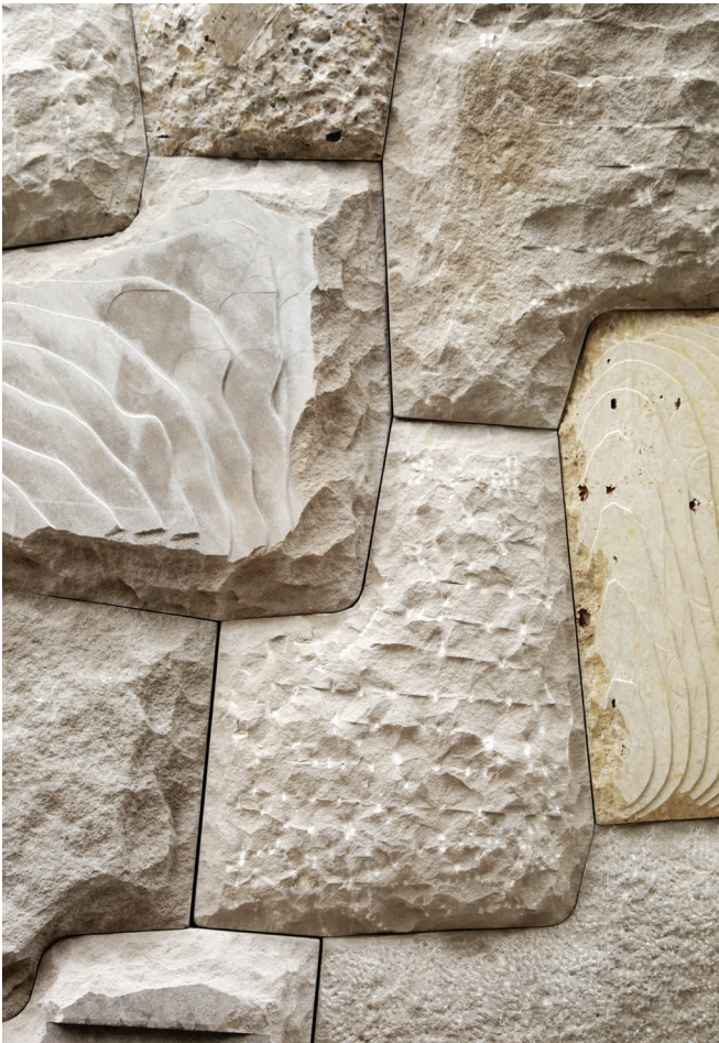
12 Detail image of the dressed front face after the manual pitching brings the stock thickness back to the intersected index edge.
